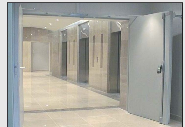
Porte battante CF 2h à 2 vantaux asservis à la détection incendie (D.A.S.). 2h Fire-Rated swinging door with 2 leaves connected to the fire detection system.
